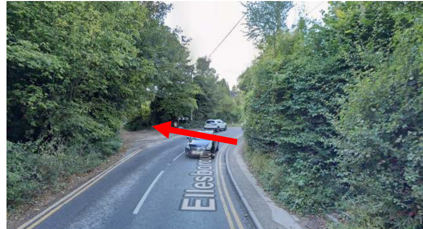
Ellesborough Road as it was
